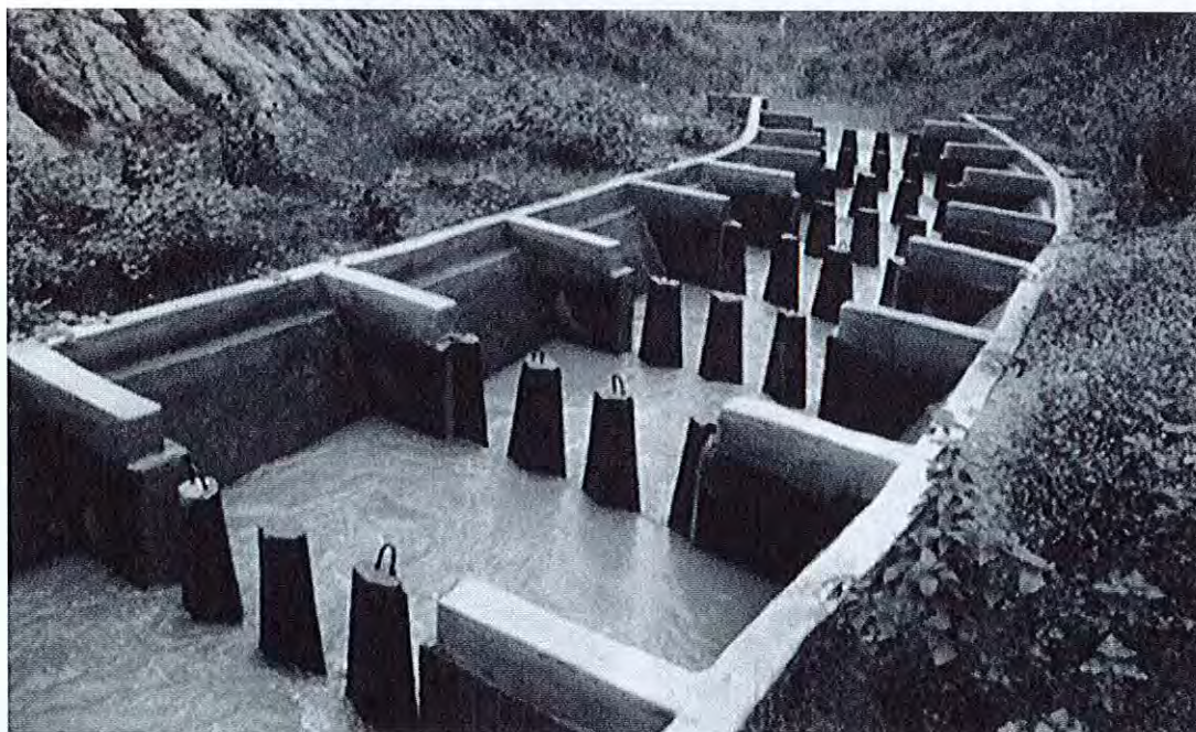
Figure 10: Example of the “cone-type” Pak Peung fishway (Lao PDR), in a tropical irrigation system. (Photo credit: Lee Baumgartner)
