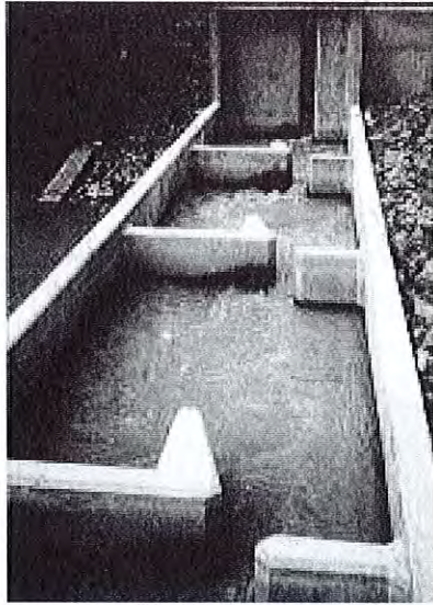
A fishway is an artificial passage of water around an obstruction in a river that enables fish to pass.
