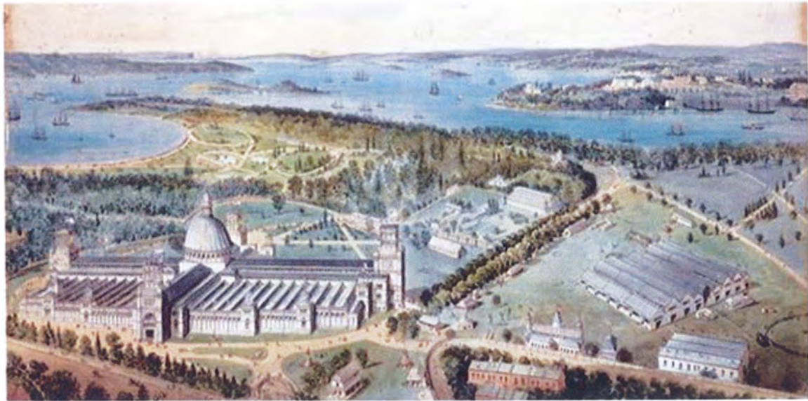
Panorama of the 1879 Sydney International Exhibition site, watercolour by John Richardson. After the disastrous fire, the Museum was re-established in the triple pitched roof building, the Agricultural Hall, bottom right corner.
