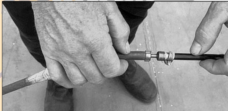
A poorly maintained welding gas supply gas line that may have leaked and caused Wu's death. Source: Media report.
