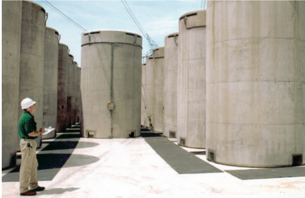
Shielding, distance and time underpins safe management of used nuclear fuel
