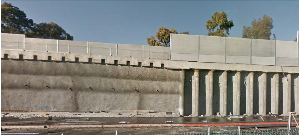
Figure 4 M5 KGR Interchange excavation under construction.
