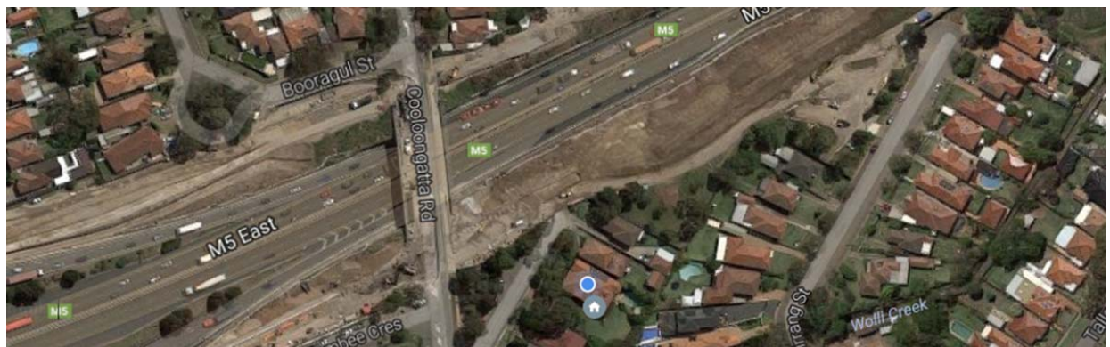
Figure 3 KGRM5 Interchange construction footprint. The blue dot represents the location of damaged buildings.
