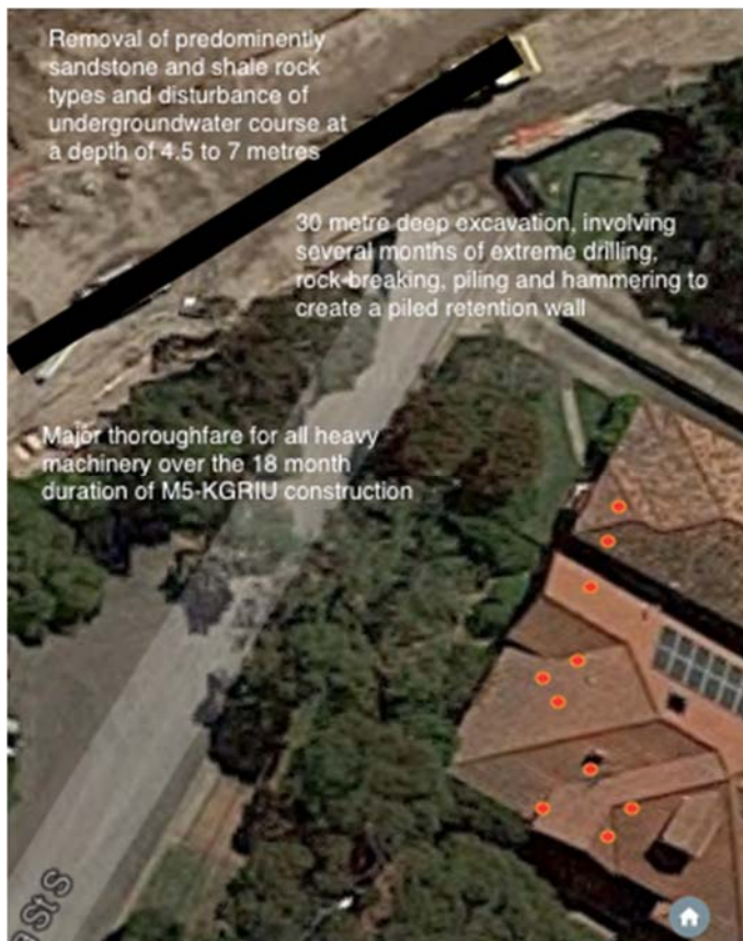
Figure 6 Pattern of initial damage through No 10 and No 8 suggesting a groundwater fault line. Damage is now extended through both homes.
