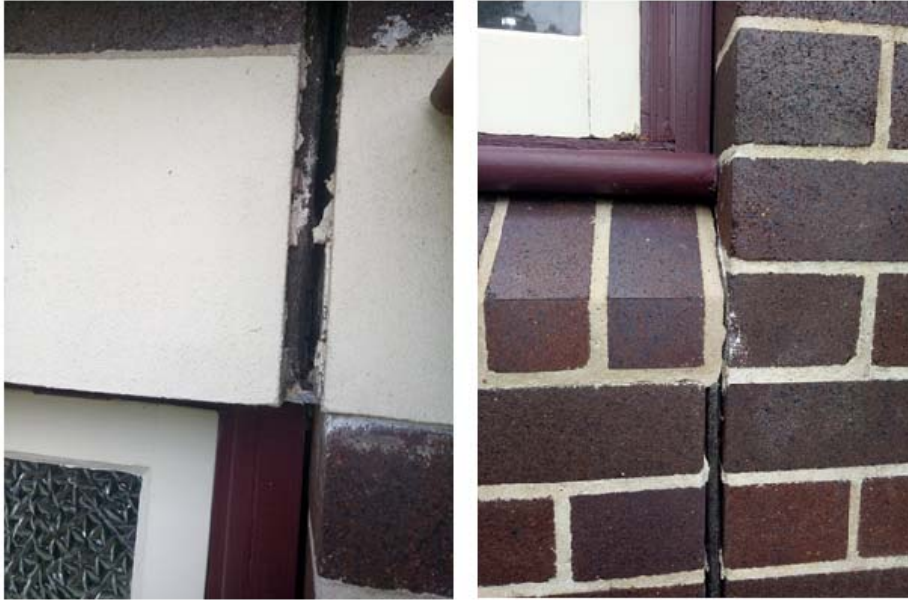
Figure 7 Separation of 1999 extension from original 1929 section
