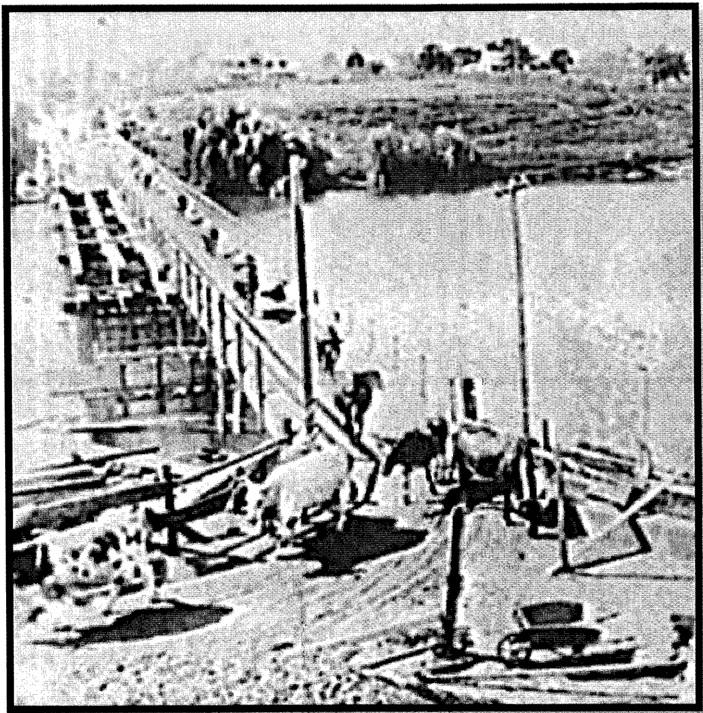
Fig 3 Bridge over Hawkesbury River at Windsor – 1922/3 - replacement of timber deck by reinforced concrete deck in half widths – note reinforced concrete beams in midground, reinforced concrete deck on beams in background
