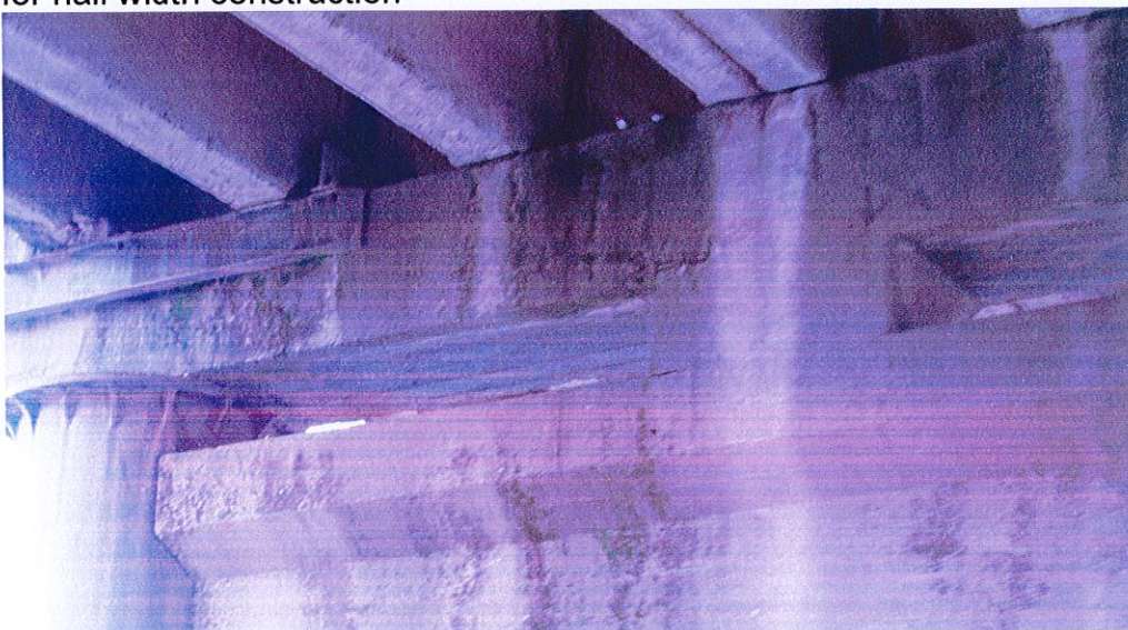
Fig 5 Windsor Bridge – note central split beam on headstock
