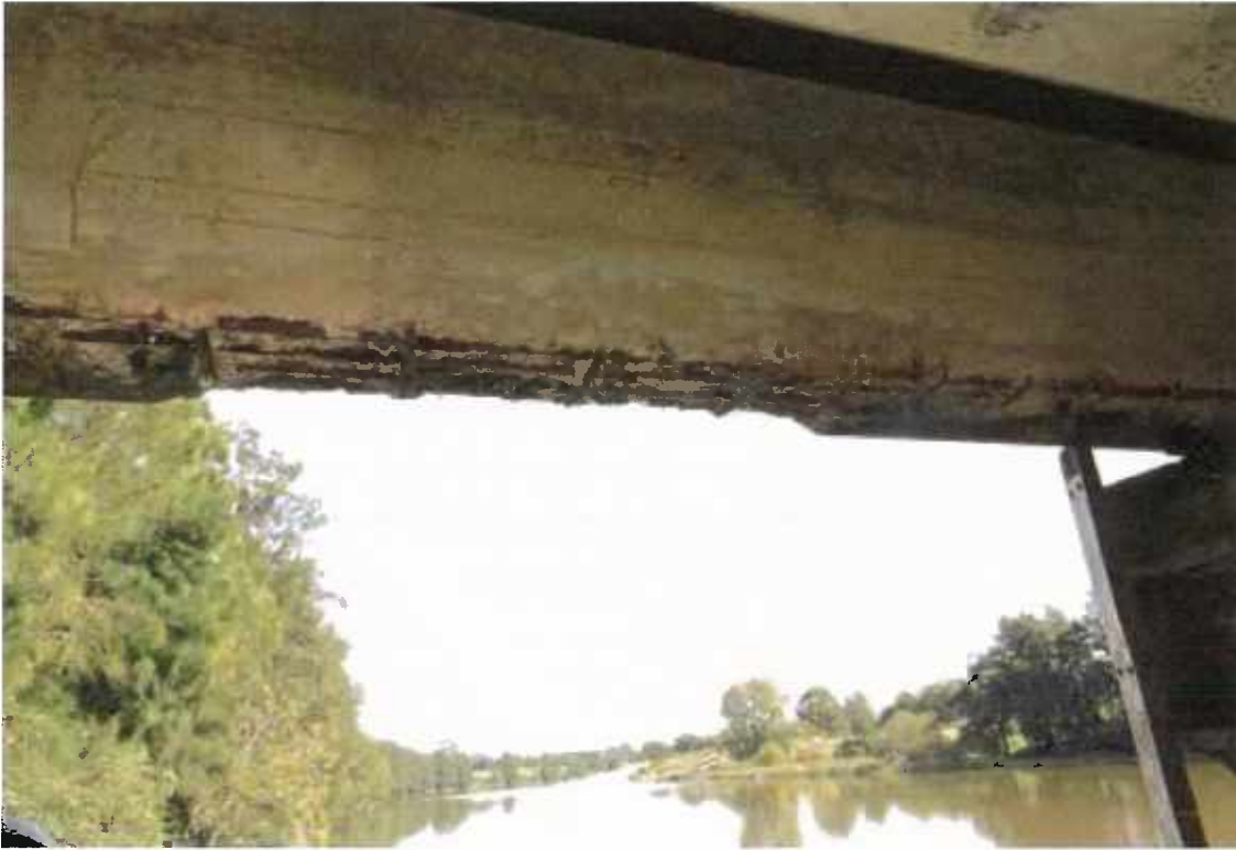
Figure 2-3 Severe spalling, delamination and corrosion of existing bridge
