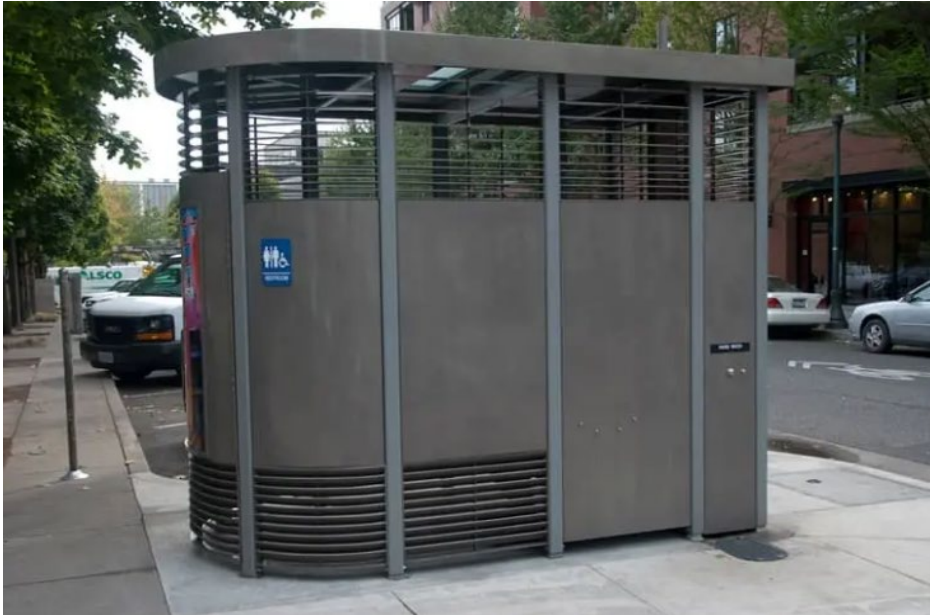
Figure 2 Photographs of the Portland Loo: 76
