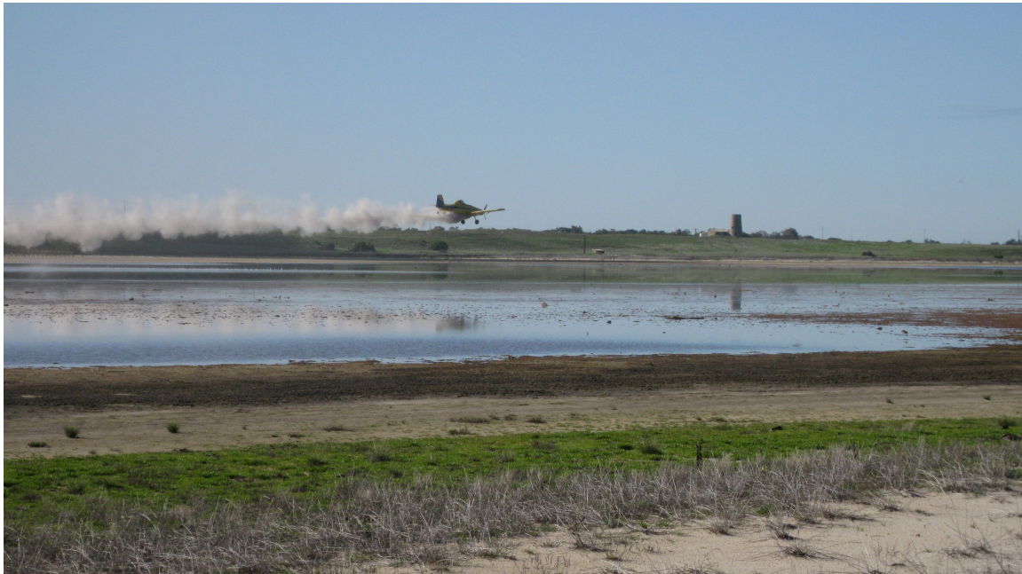
Liming highly acidic water and acidic soils exposed in Currency Creek that flows into the Goolwa Channel. Pix by Ken Jury.
