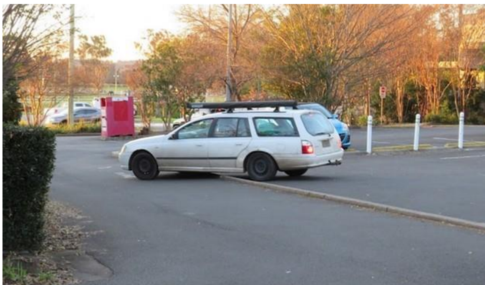
Photo 1: Vehicle travelling over rollover kerbing
