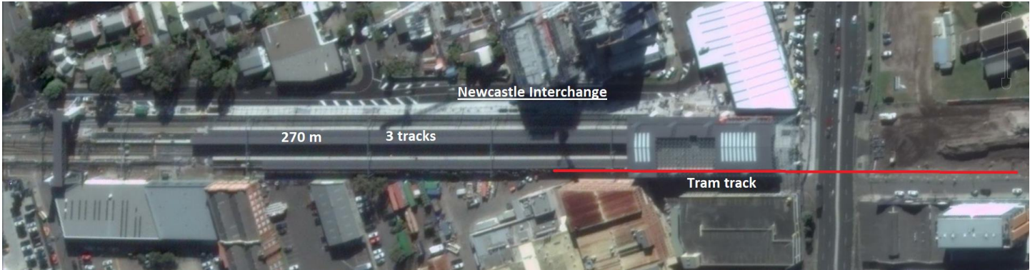
Newcastle Interchange – requires tram track for completion
