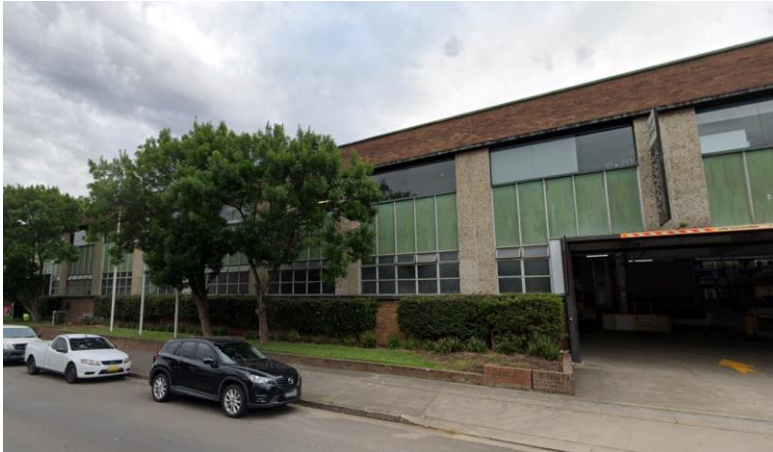
Figure 2 – Carnarvon Street view (Google maps September 2023)
