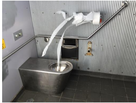
Figure 10: Wattaka Rest Areas, Hunter Expressway
