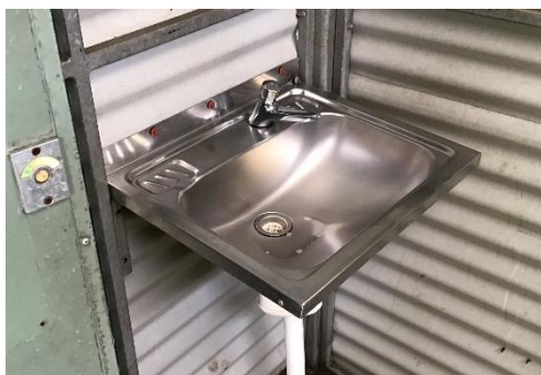
Figure 8: Gowan Rest Area S/B, Newell Highway
