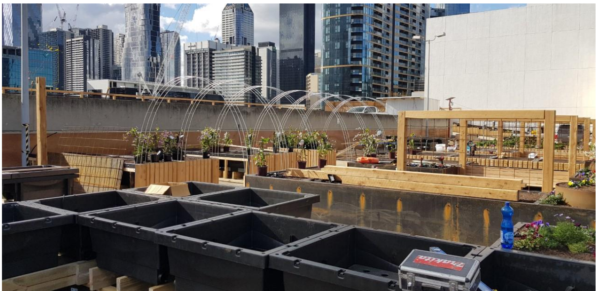
Figure 8: Wicking-beds being built to incorporate seating and dining areas.
