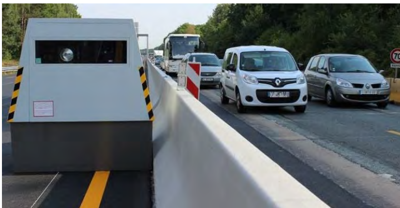
Figure A.26 France: Autonomous temporary speed camera commonly used at worksites in France.
