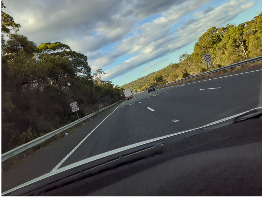
Faded 110 km/hr road markings (been like this for many years). Ironically it is located just 500 metres past a fixed speed camera. Location: M1 northbound Bar Point NSW
