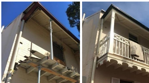
Figure 19: End balcony during and after replacement
