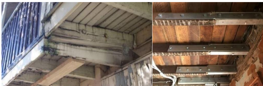
Figure 19: End balcony during and after replacement
