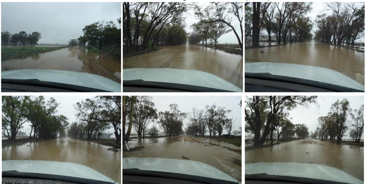
IR final alignment - Wallaby Rd 5 th March 2020 – 65 mm of rain in 24hr Minimum 5km of this section of the alignment inundated up to depth of 40cm
