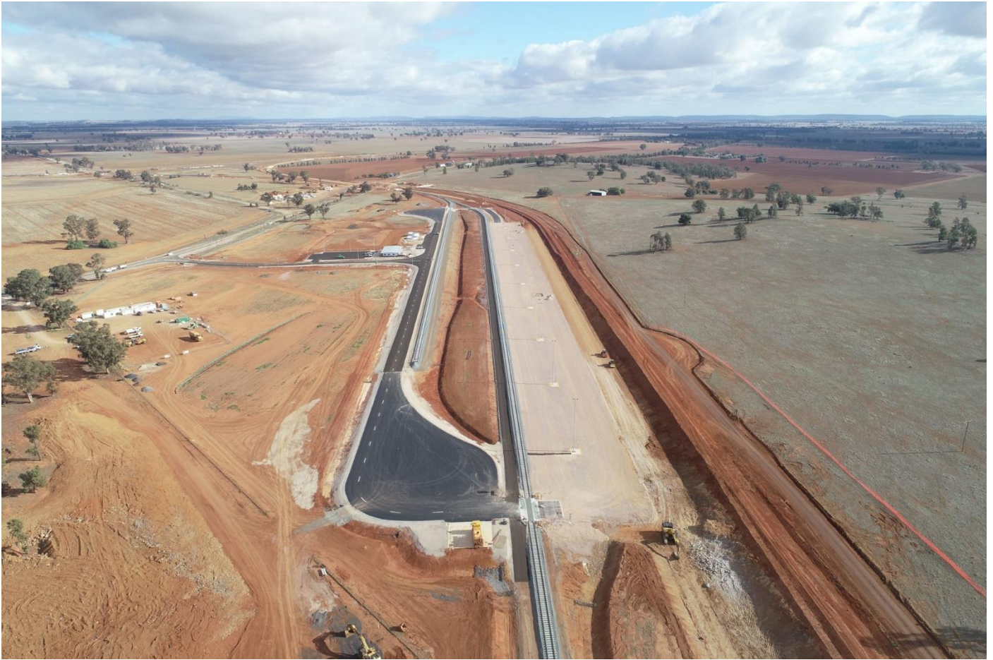
Pacific National Intermodal terminal under construction 2019
