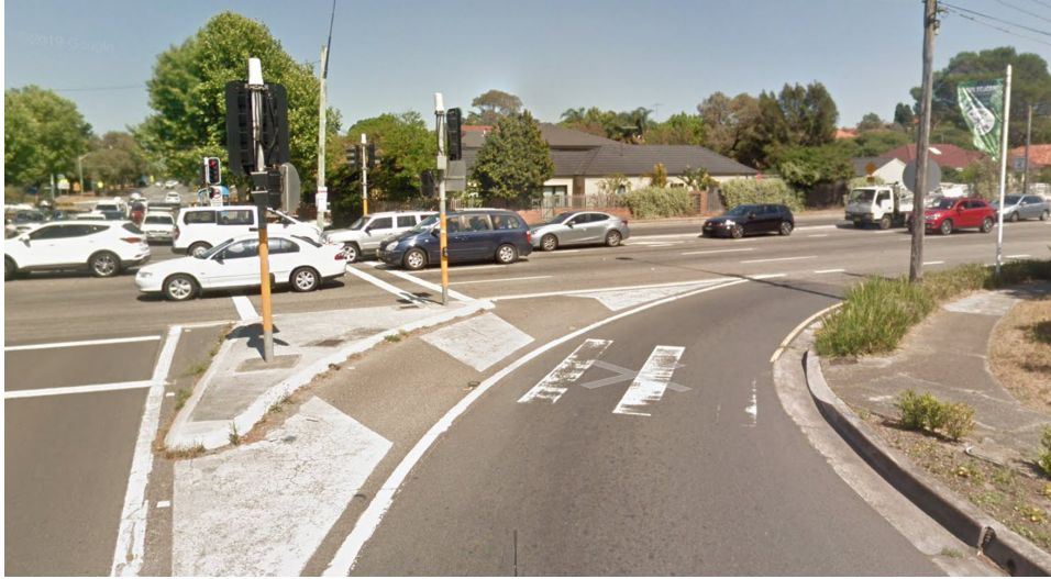
Wentworth Ave / Page St Pagewood. 3 way refuge island has no kerb ramps, requiring people to pause or stand on the roadway. Wentworth Ave is signposted 70km/h.
