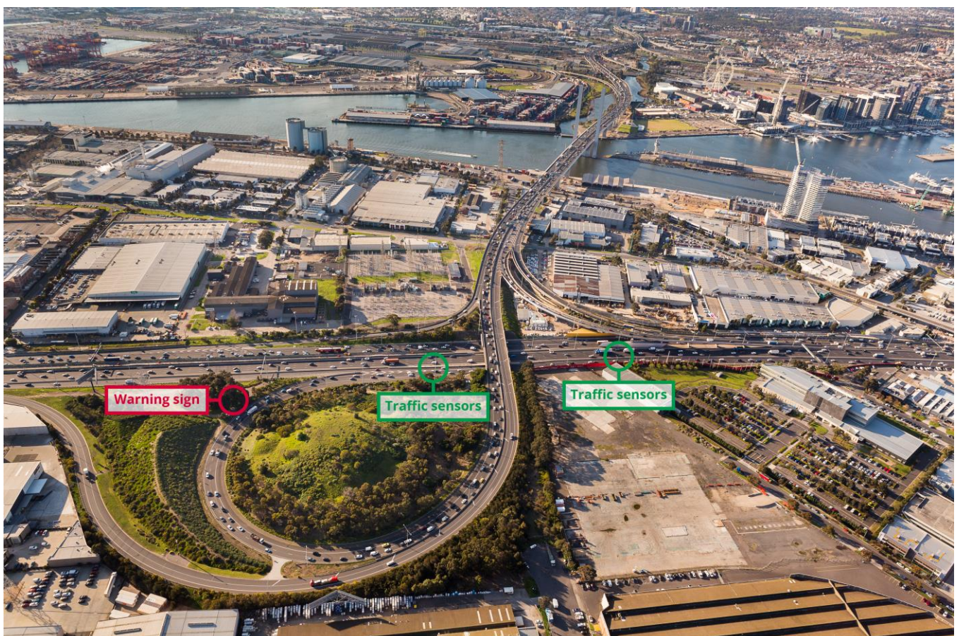
Figure 2 – Westgate Freeway and Bolte Bridge interchange
