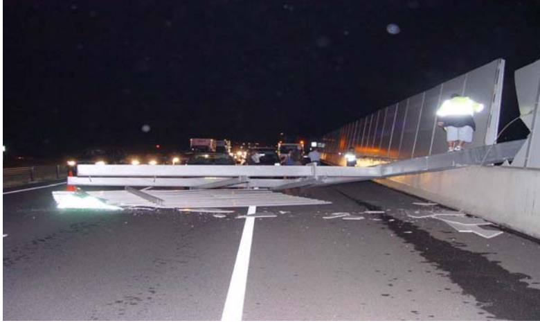
Photo 1 Bolts failure
