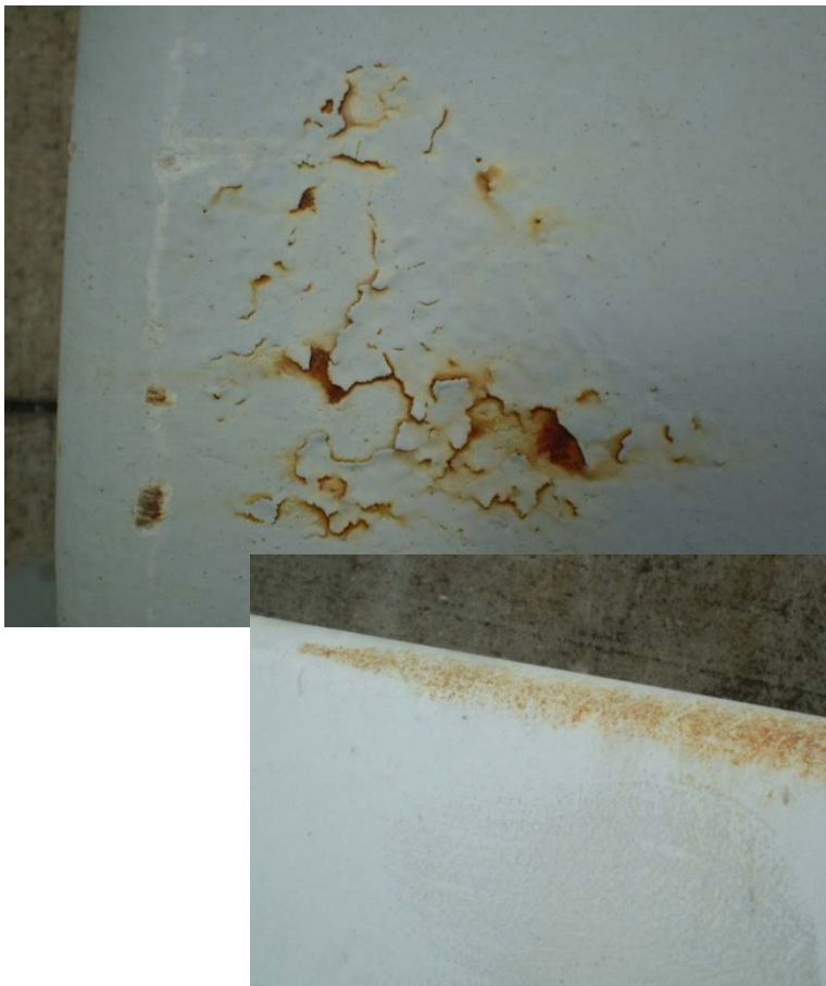
Photos 5-6 Poor paint finish against a specification of 75um inorganic zinc silicate, 6. 125um epoxy and 75um urethane. Top coat left off.
