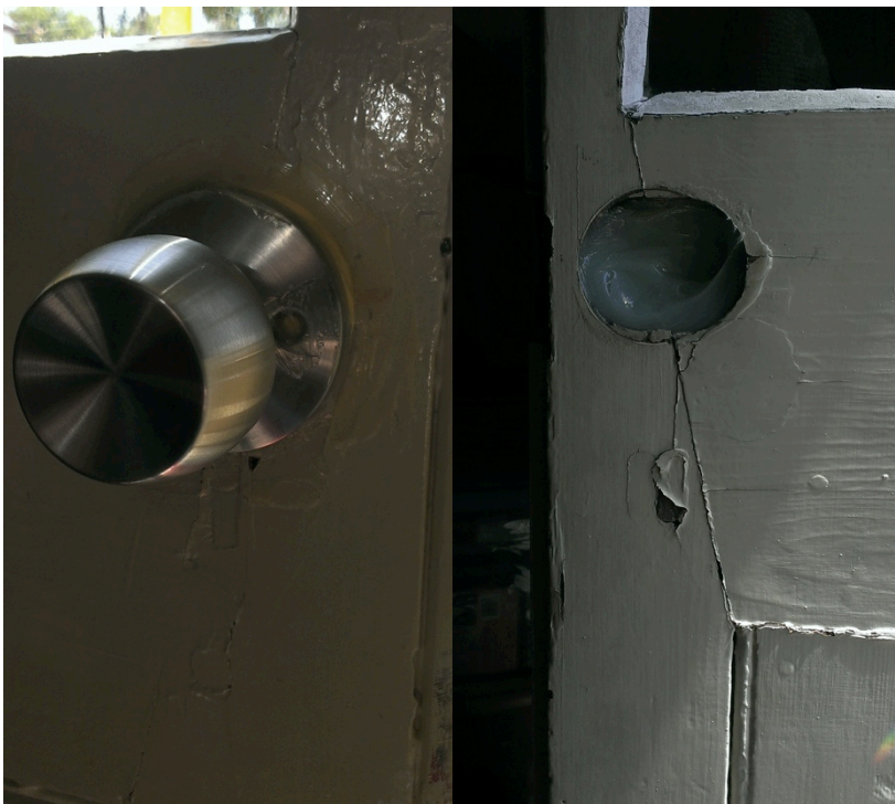
Interior Knob and on the exterior - just a glob of glue.
