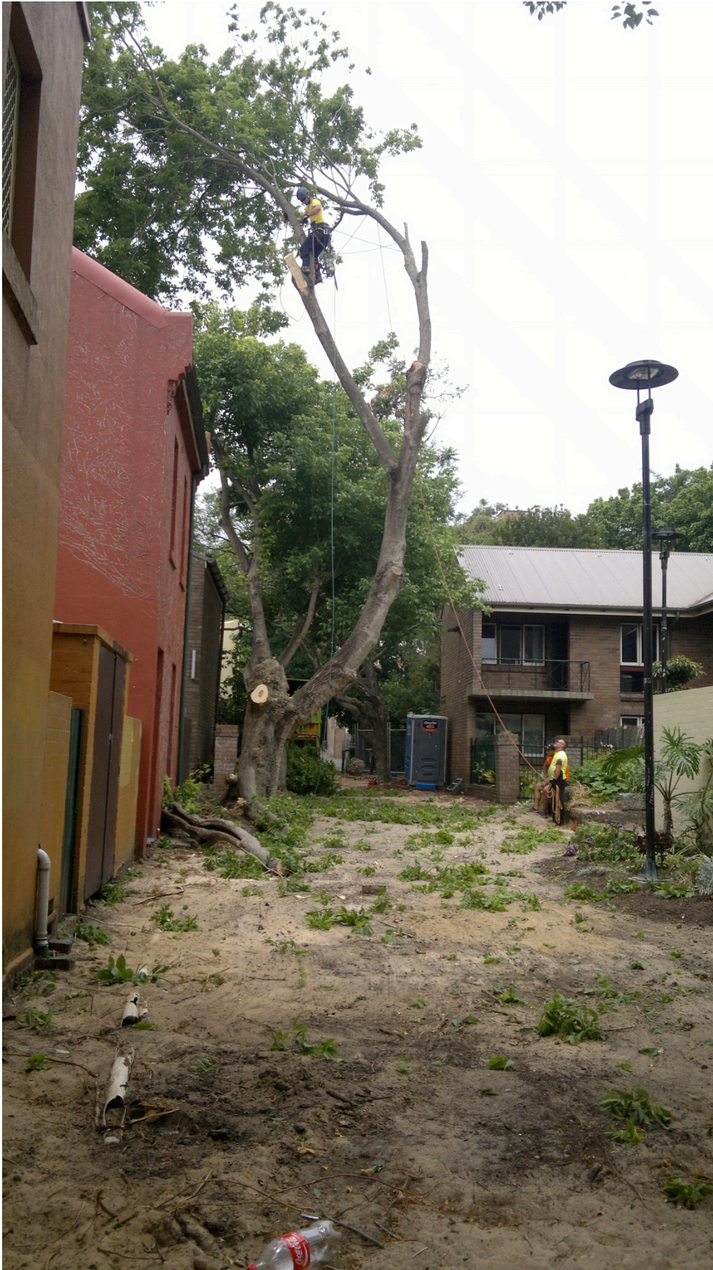
Stephen St with pavers removed and tree removal Nov 2015
