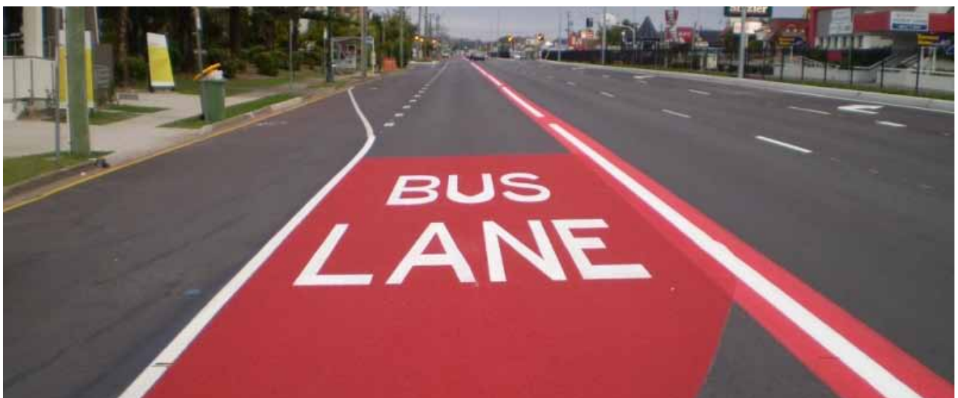
Figure 14: Example of painting only the start of the bus lane in red, and also painting the line separating the bus lane from the adjacent traffic lane. Brisbane City Council has adopted this approach. Source: Safe T Surfaces (STS) www.safetsurfaces.com.au
