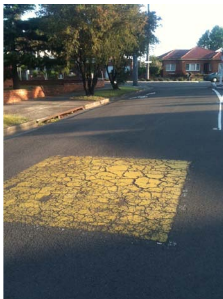
Figure 11 – photograph of a deficient 40km/h school zone 'patch' at Bardwell Park in Sydney's south (October 2011).
