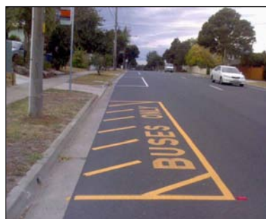
Figure 3 – example of pavement markings used in Victoria to deter illegal parking and assist public transport
