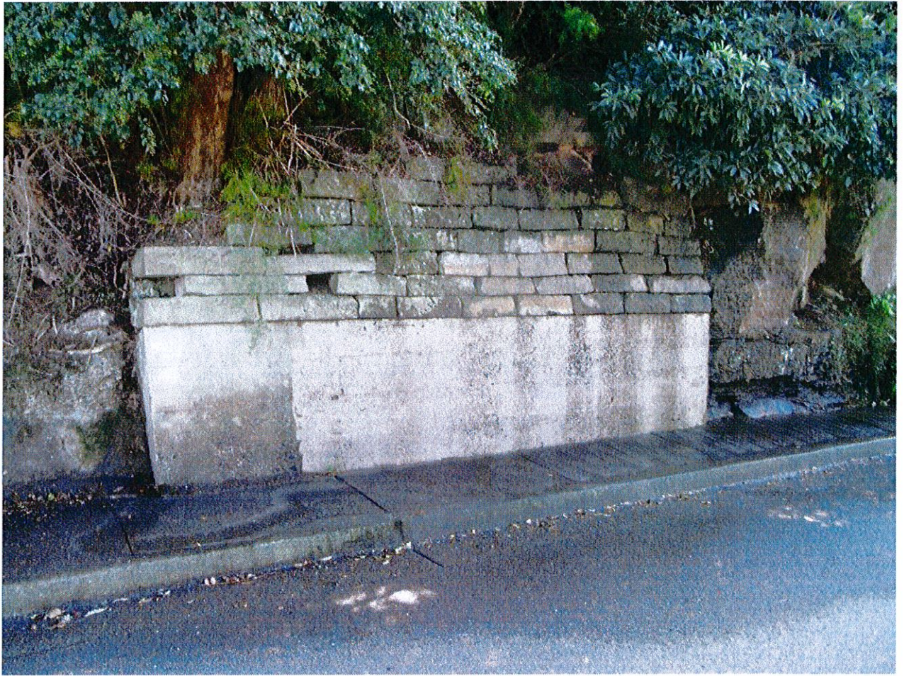
As cleaned by Gurney – most effective method on stone concrete and unpainted surfaces.
