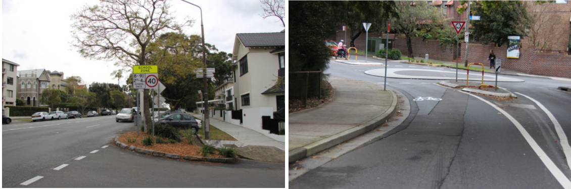
Poor visibility due to roadside furniture and signage, the signs can hide a car let alone a bike.
