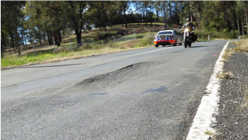
Putty Road, ridge in centre of lane at exit of bend, firmly placed in the line of travel for a motorcycle.
