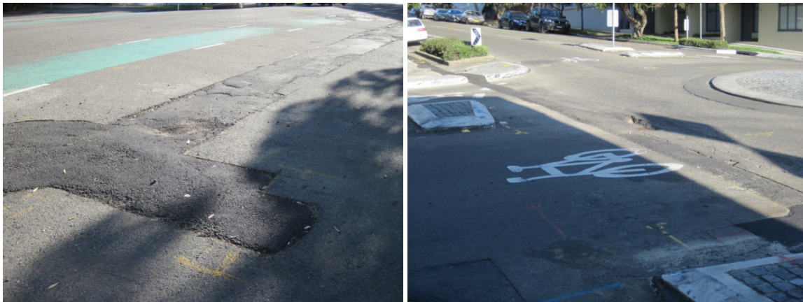
Poor road repair in braking areas on approaches to Collins St.
