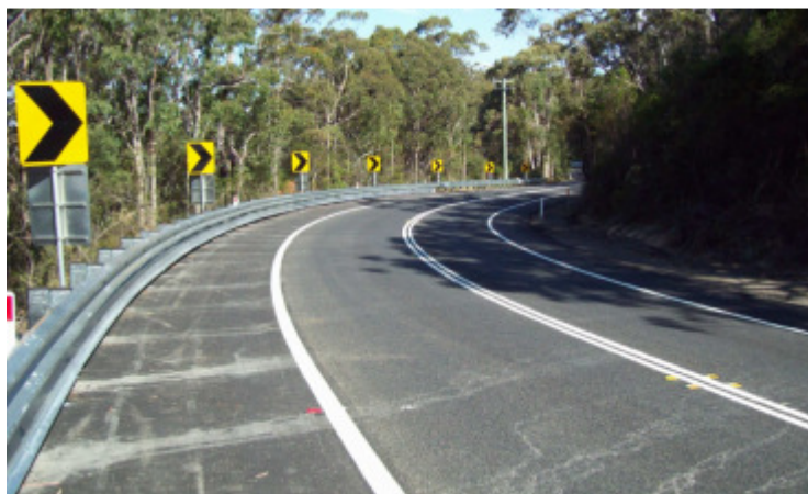
Installation of under run/rub rails on W Beam barrier on the Old Pacific Highway
