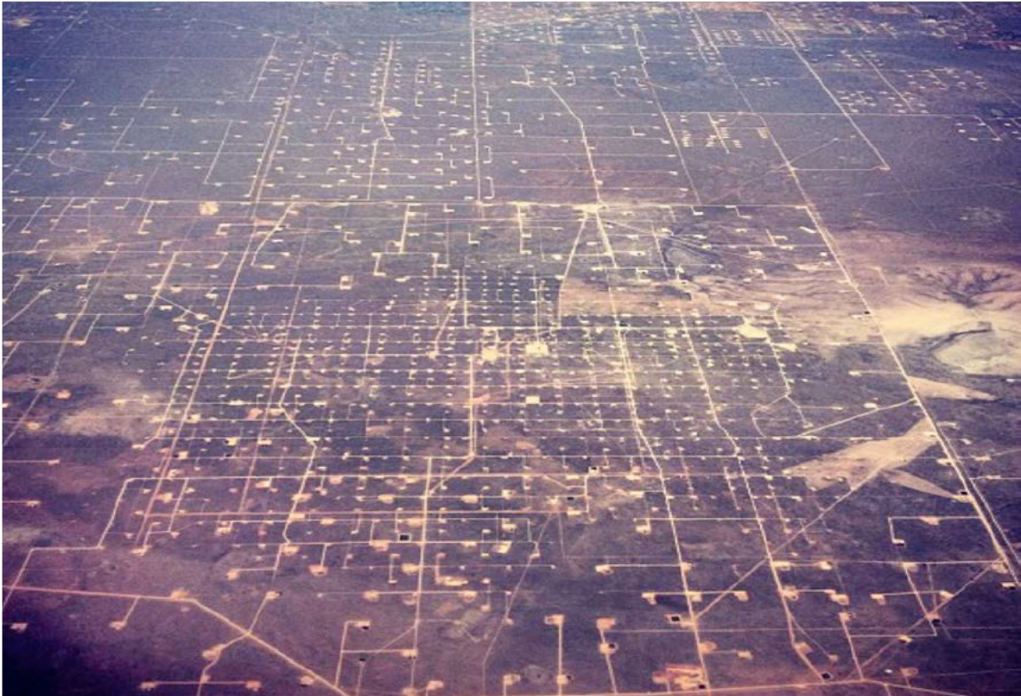
A coal bed methane (CSG) field in the United States shows clearly the degree of industrialization required.
