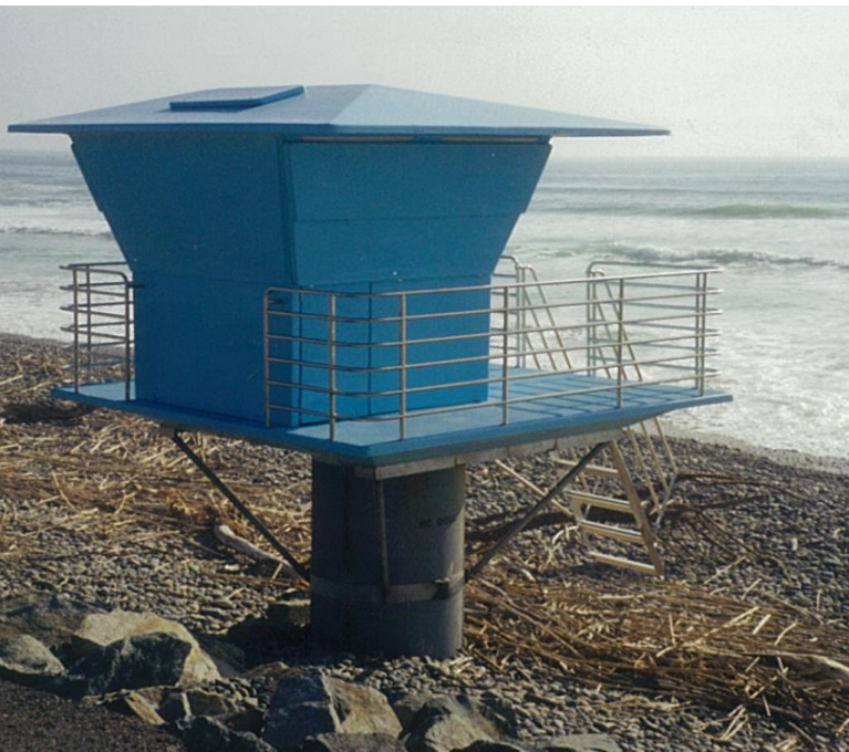
Permanent pillar foundation for hurricane prone areas
