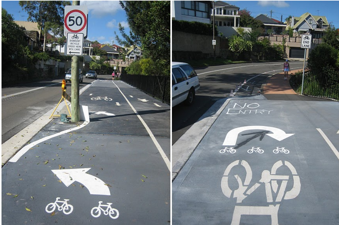
This signage at Henley Marine Drive, Drummoyne directs bicycle riders to cross the road to avoid the end of cycle path ahead. A ramp is hidden behind the power pole. There is no signage to direct bicycle riders whether they should continue along the main road or take a side street. At the end of the cycle path, bicycle riders are directed to make a u-turn. This is a popular recreational route and provides access to Birkenhead Shopping Centre. Photos: Robert Moore
