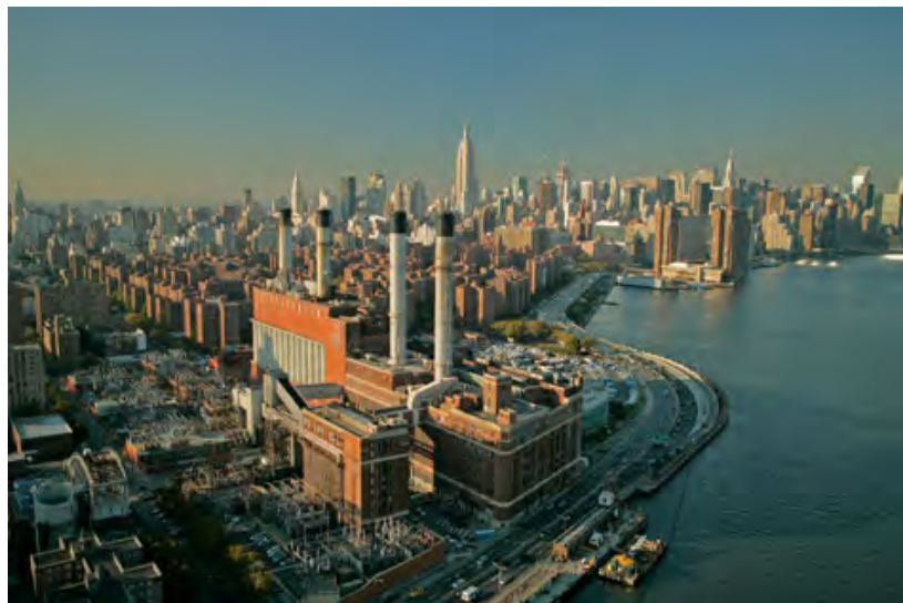
Figure 12 – Con Edison 15 th Street Cogeneration Plant
