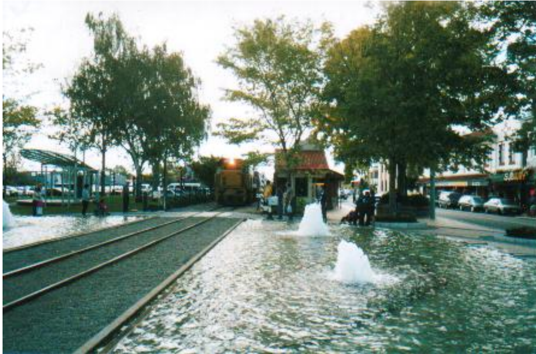
Figure 5 - Water features incorporated into rail corridor in Hastings, NZ
