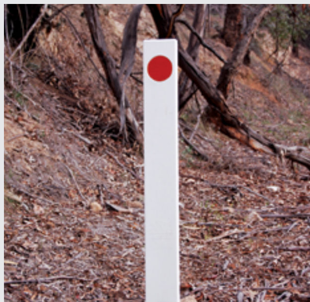
Use of motorcycle friendly (frangible when hit by a rider or pillion) guide posts can improve safety.
