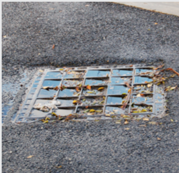
Steel utility covers can present a very slippery surface to a motorcycle or scooter.
