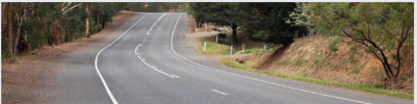
Sealed road shoulders can provide additional safety for motorcycles, scooters and other vehicles.
