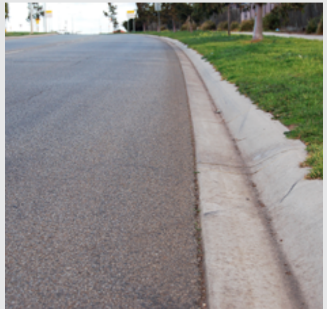
Semi-mountable kerbing reduces the likelihood of a crash if ridden over by a motorcyclist.
