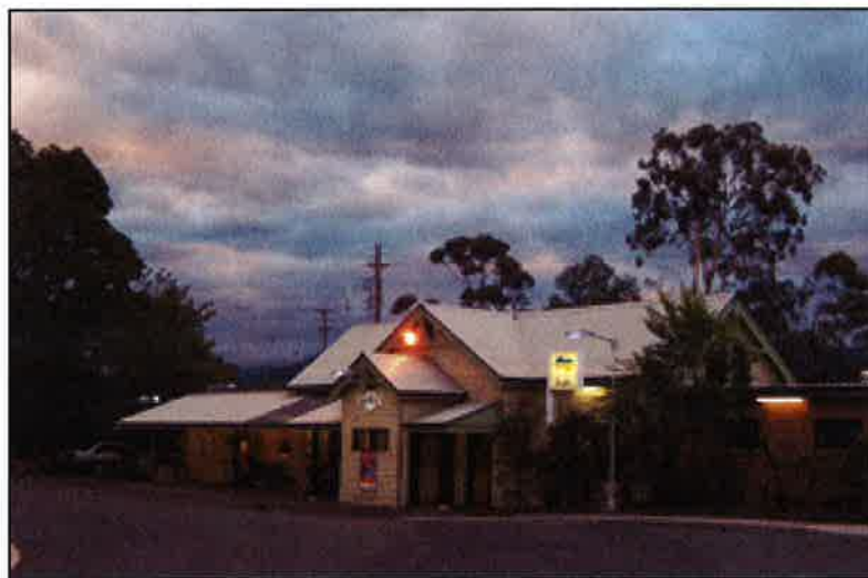
Figure 8. Dapto Railway Station Entrance (existing)
