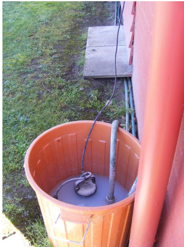
FIGURE 3: COLLECTION AND STORAGE OF UNTREATED GREYwater FOR IRRIGATION
