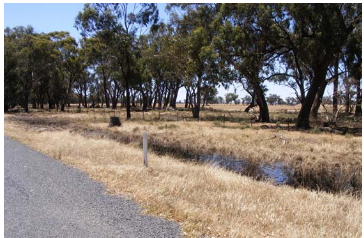
Forbes - 12 th December, 2009 Irrigation water spilling into table drains for 100's metres
