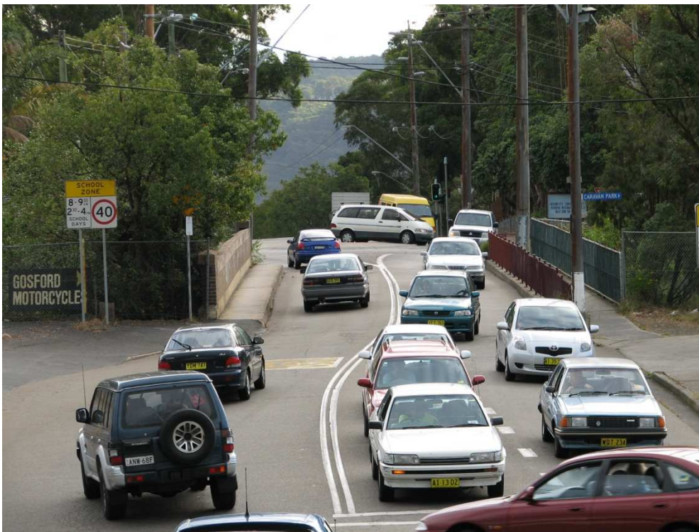
Etna Street rail overbridge looking west showing inadequate footway/ cyclist/ traffic areas
