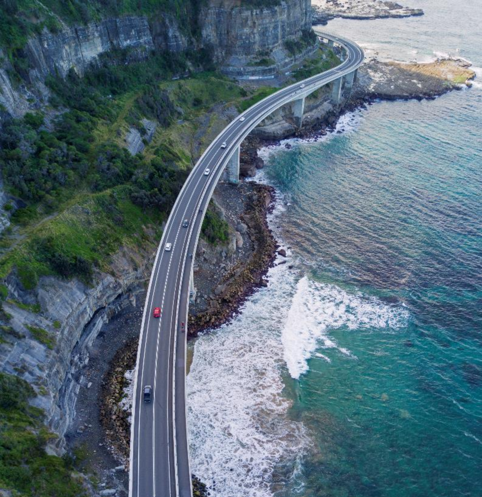
Sea Cliff Bridge, Wollongong
