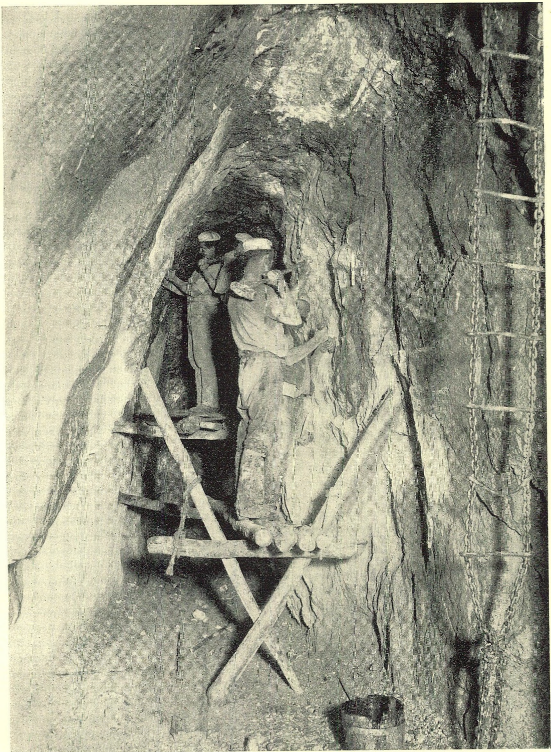
"WENTWORTH PROPRIETARY" GOLD MINE, LUCKNOW, N.S.W. (Miners engaged in over-hand stoping.)
