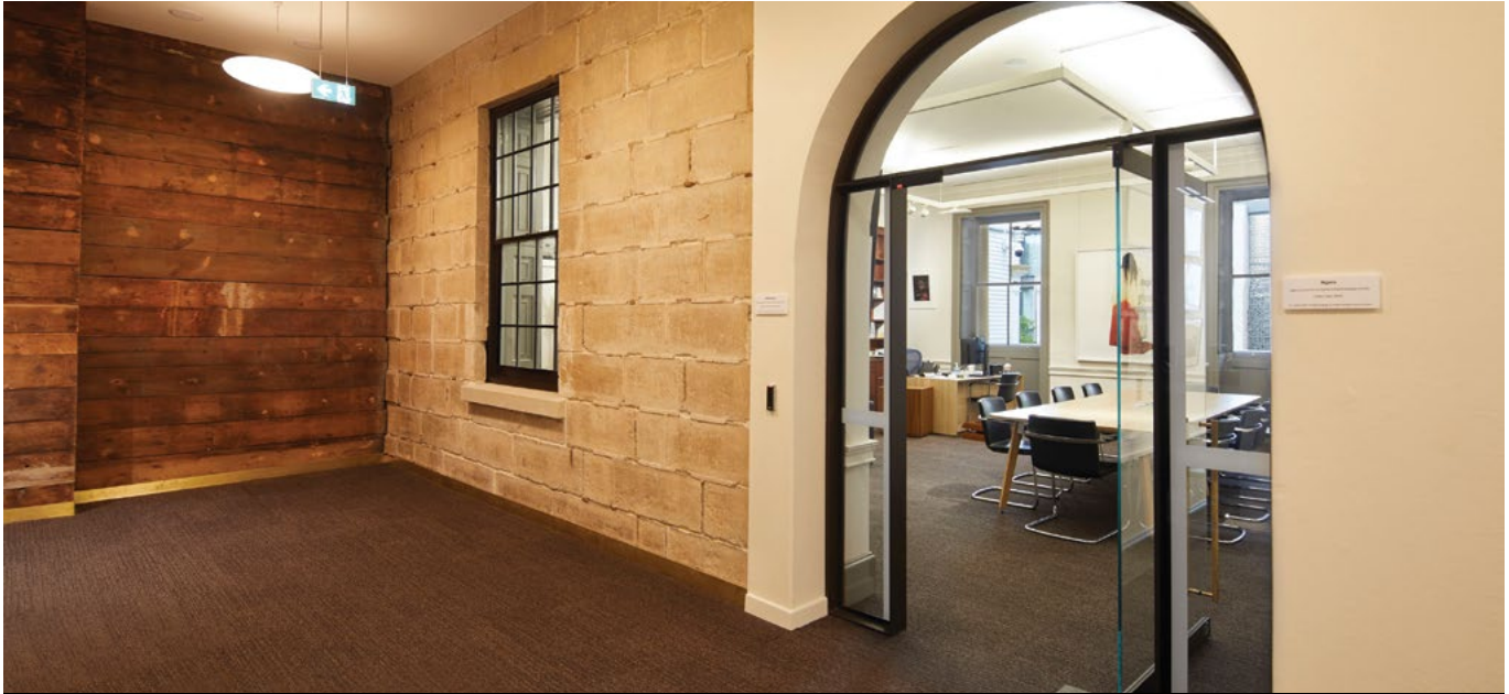
Capital Works team managed the refurbishment which revealed heritage features including the original timber wall
