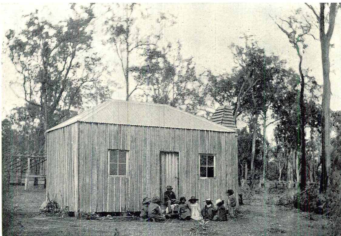
HOUSE BUILT FOR JACK TORRENS BY HOME STAFF, GRAFTON.
