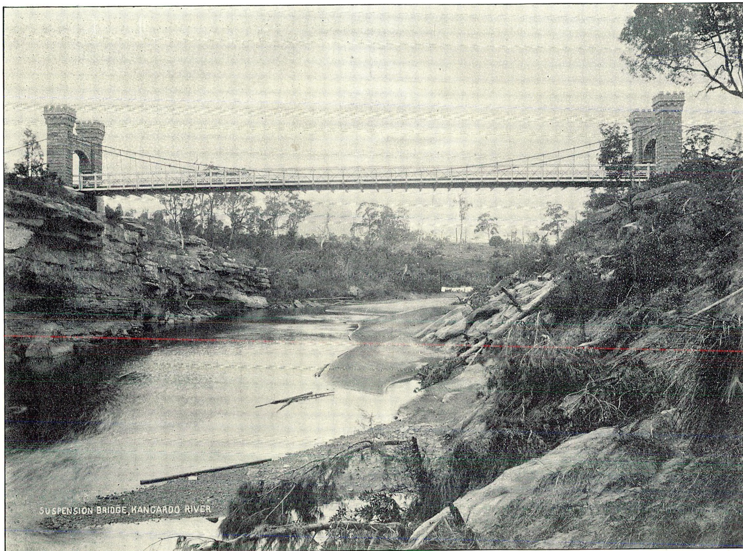
HAMPDEN BRIDGE, OVER KANGAROO RIVER, ON MOSS VALE-NOWRA ROAD. Span, 252 ft. 9 in. Width of Carriage-way, 18 ft. Height of Deck above Summer water-level, 63 ft.
