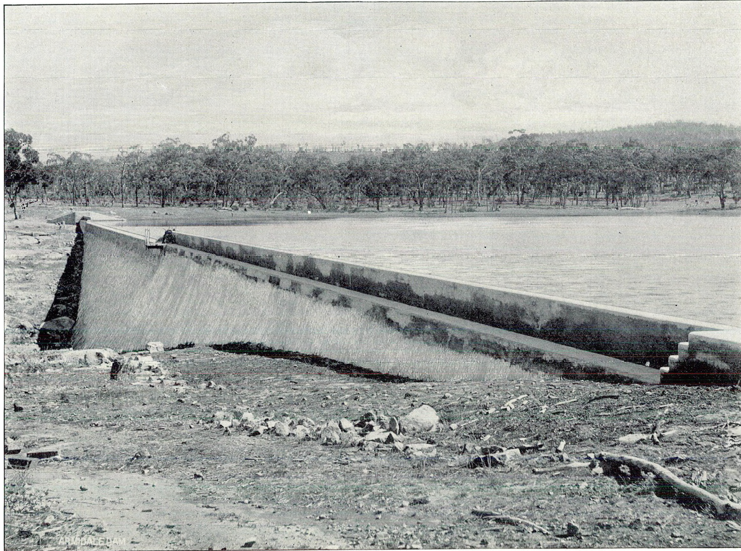
ARMIDALE DAM ARMIDALE WATER SUPPLY—CONCRETE DAM AND STORAGE RESERVOIR.
