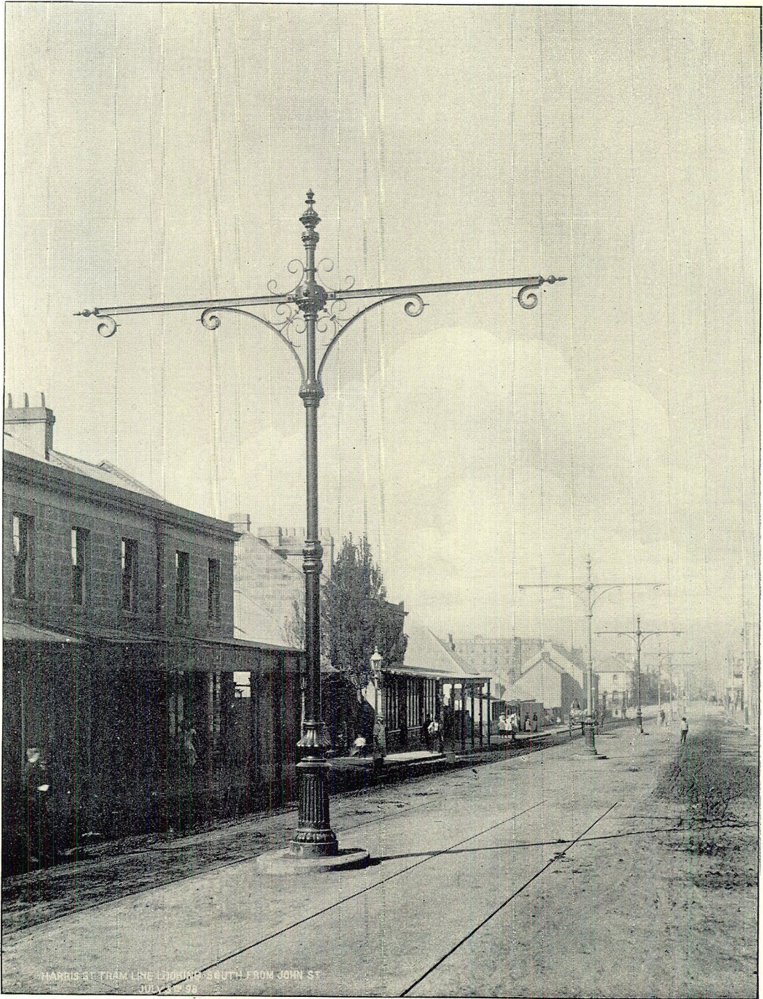
GEORGE-STREET AND HARRIS-STREET ELECTRIC TRAMWAY. View in Harris-street, showing Mannesmann Poles and Brackets.
