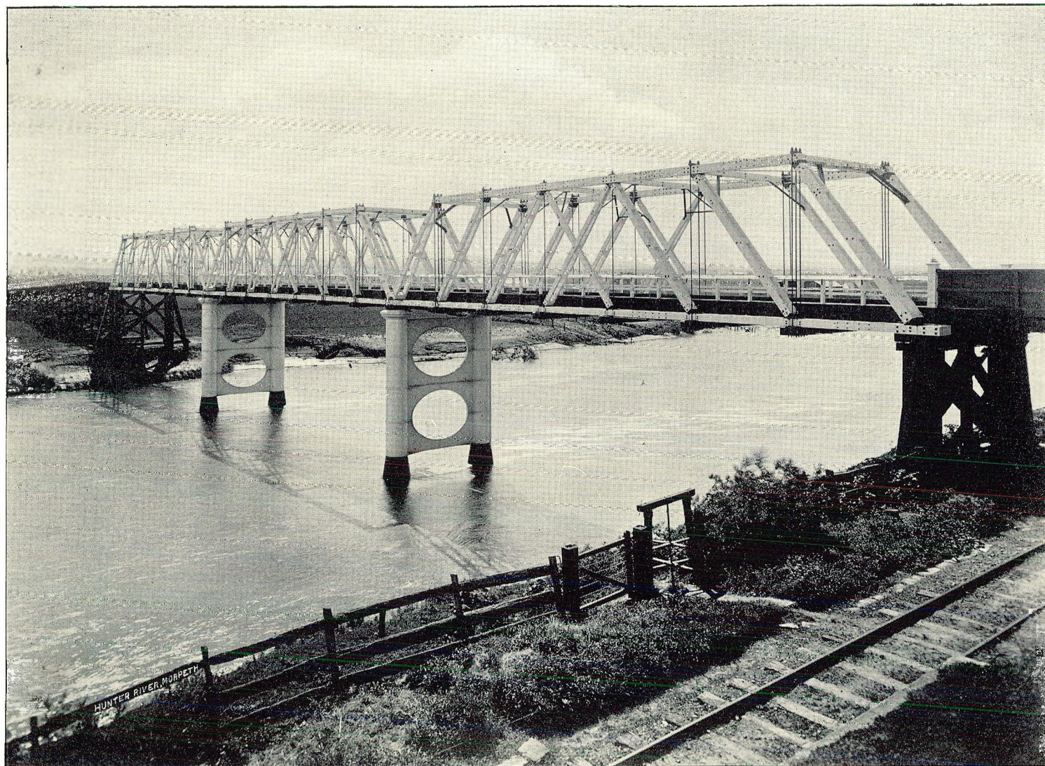
MORPETH BRIDGE, OVER THE HUNTER RIVER, AT MORPETH. Length, 819 ft. Width of Carriage-way, 18 ft. Height of Deck above high-water level, 36 ft. 6 in.
