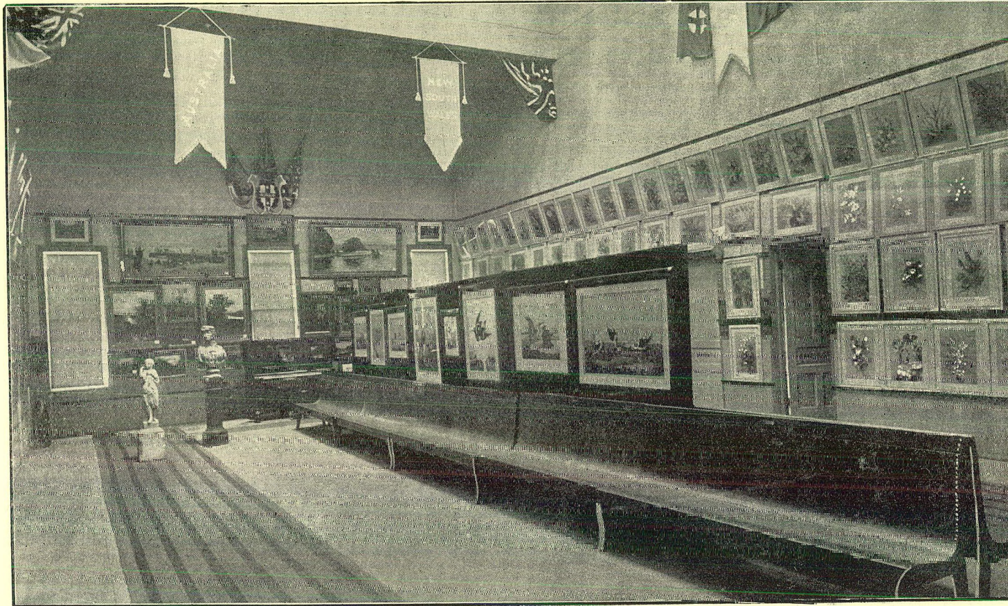
HALL, "AUSTRALIA HOUSE," NEW SOUTH WALES ADMINISTRATIVE BUILDING.
