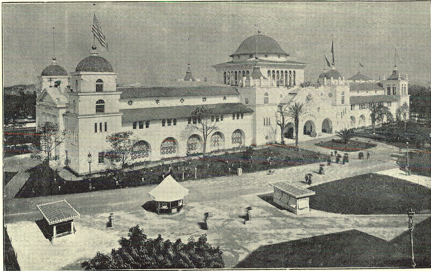
CALIFORNIA STATE BUILDING.
