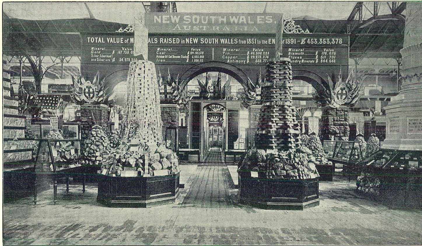
NEW SOUTH WALES COURT, MINES BUILDING, TRANSVERSE VIEW.
