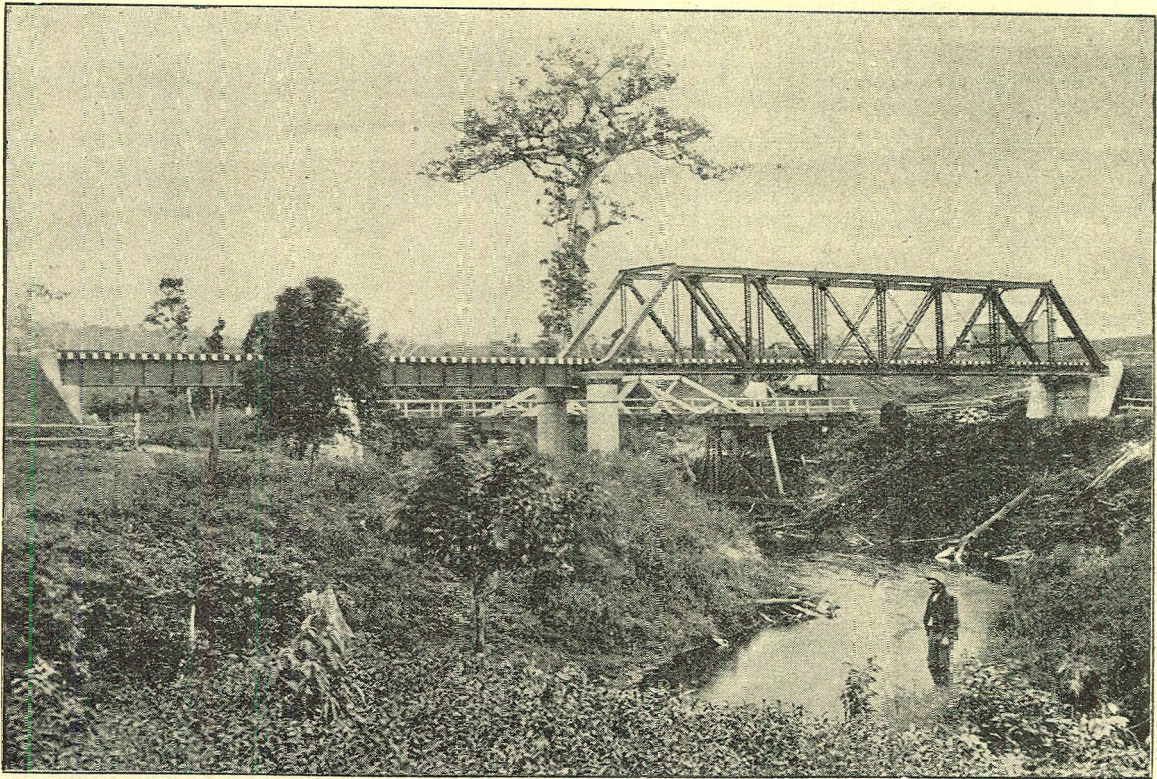
NO. 4.—BRIDGE OVER WILSON'S CREEK, LISMORE TO THE TWEED RAILWAY.
